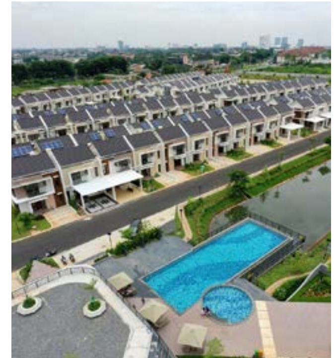
Foto: Panel Surya di Klaster Burgundy Resident, The Orchard, Summarecon Bekasi
